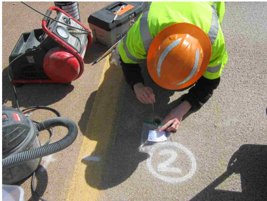
Figure 3-5: Concrete sampling for chloride concentration analysis.
