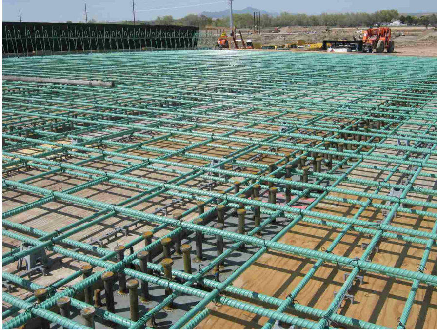
Figure 2-5: Epoxy-coated reinforcement.
