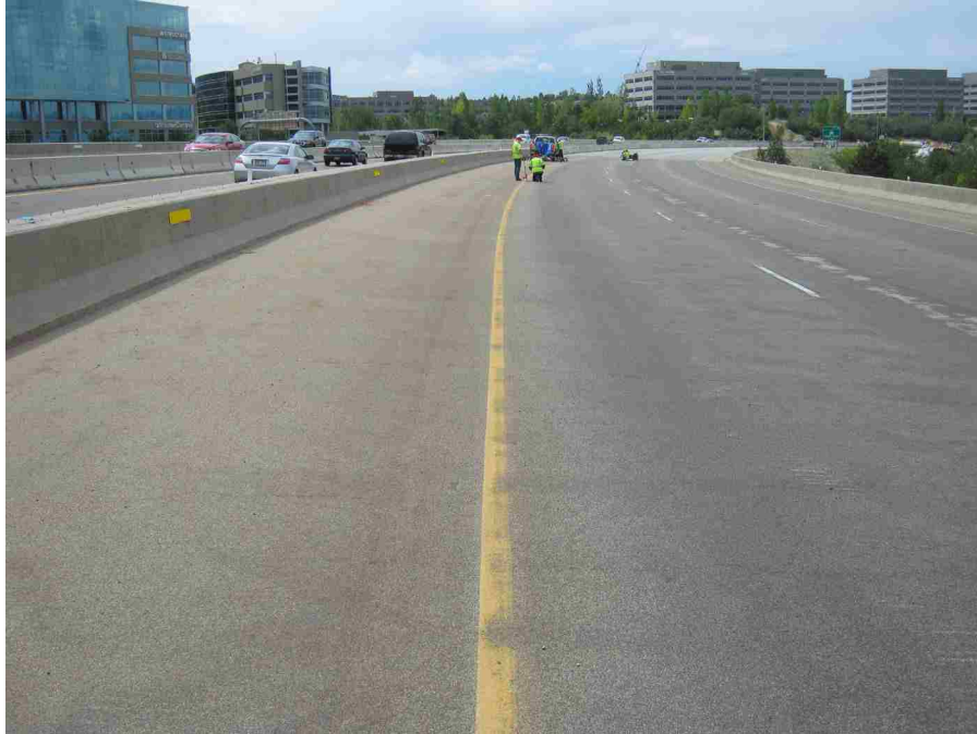
Figure 2-7: Deck with polymer overlay.
