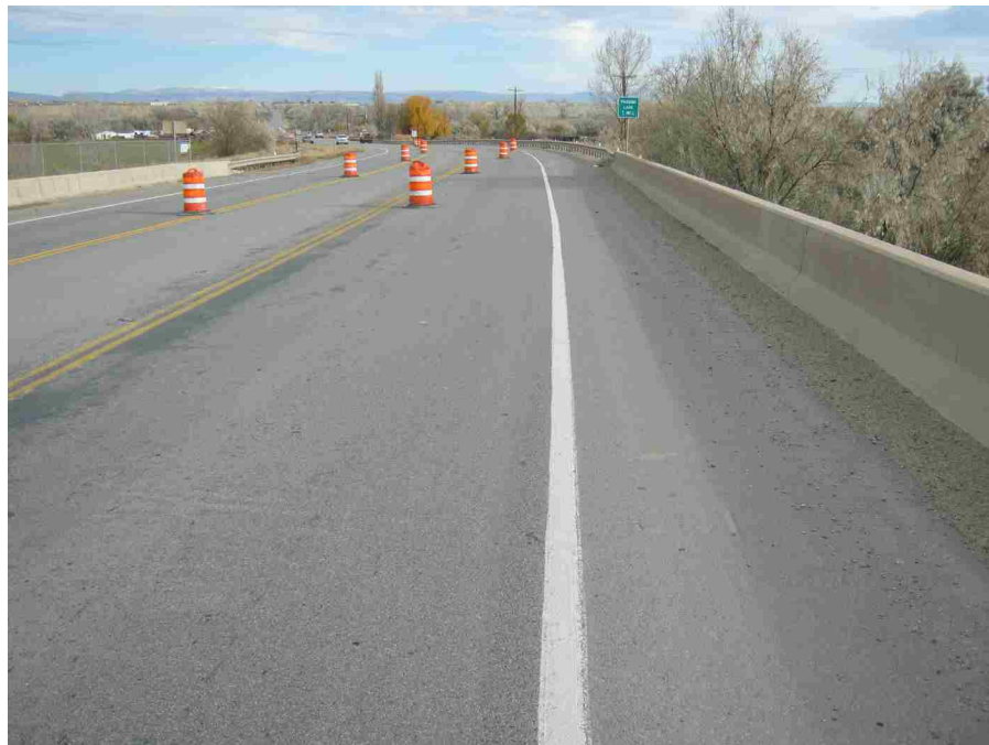
Figure 2-6: Deck with asphalt overlay.
